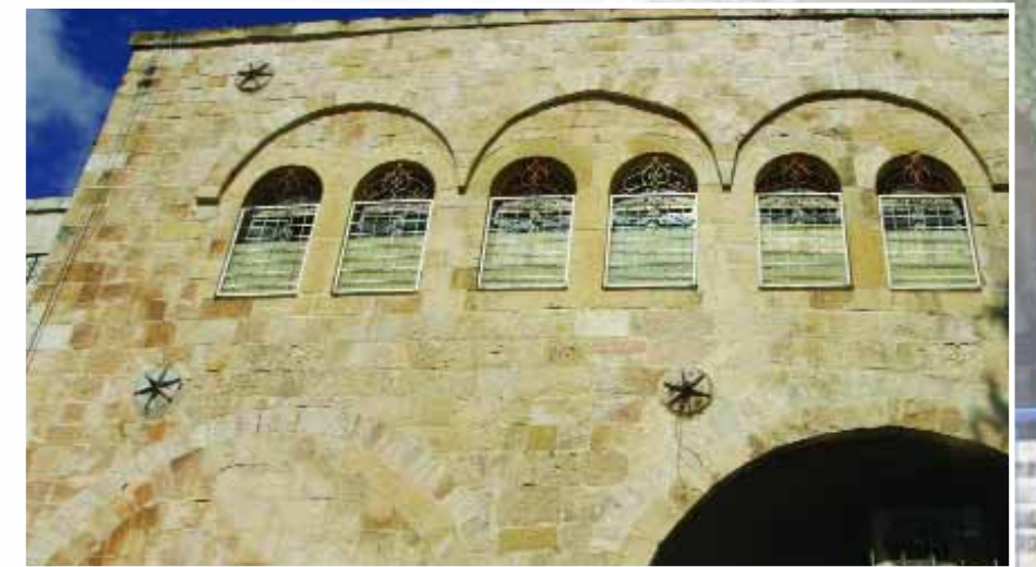
The yeshivah ketanah building
